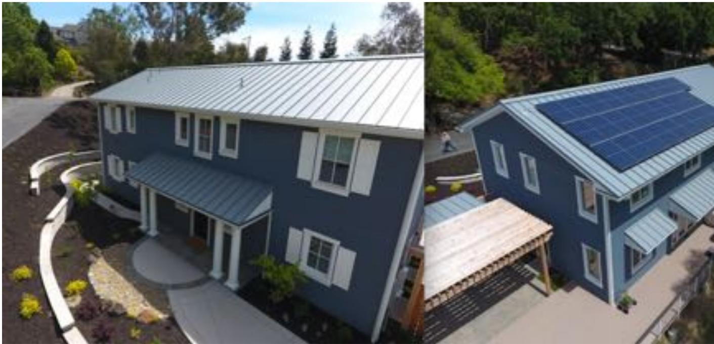
*Figure 9 composite: Alamo Passive House by One Sky Homes is an all-electric home. The project includes a 7.5kW PV array on the south-facing roof that generated 12,767 kWh of energy to offset a net annual energy use of 10,707 kWh by the house and electric vehicle.*
